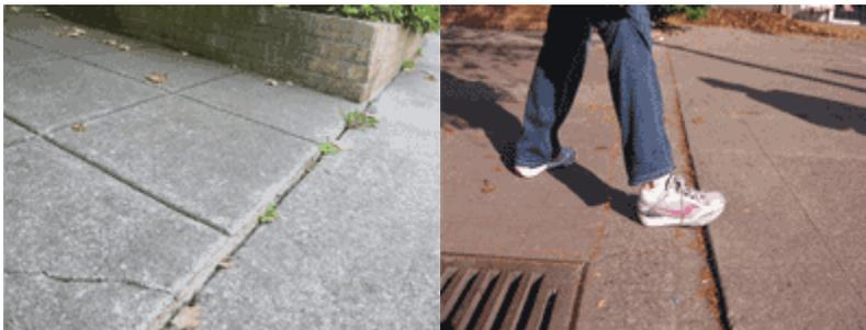
**See two other issues: a tripping hazard created where grade of sidewalk and private property are not aligned and two different types of surface treatments can result in tripping hazard over time.**
