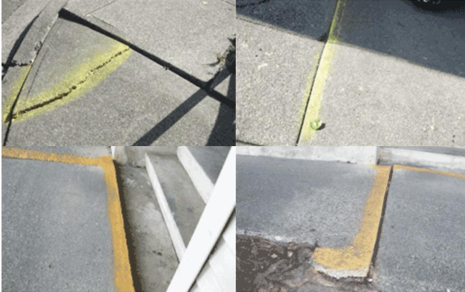
**Pictures of barriers to walkability in Ladner Village. The first two pictures are of cracks in the south side of Bridge Street, west of Elliot. Sidewalk and entrance to building not at same grade on Bridge Street. In fourth picture see how a tree root lifts the sidewalk and expands the sidewalk crack.**
